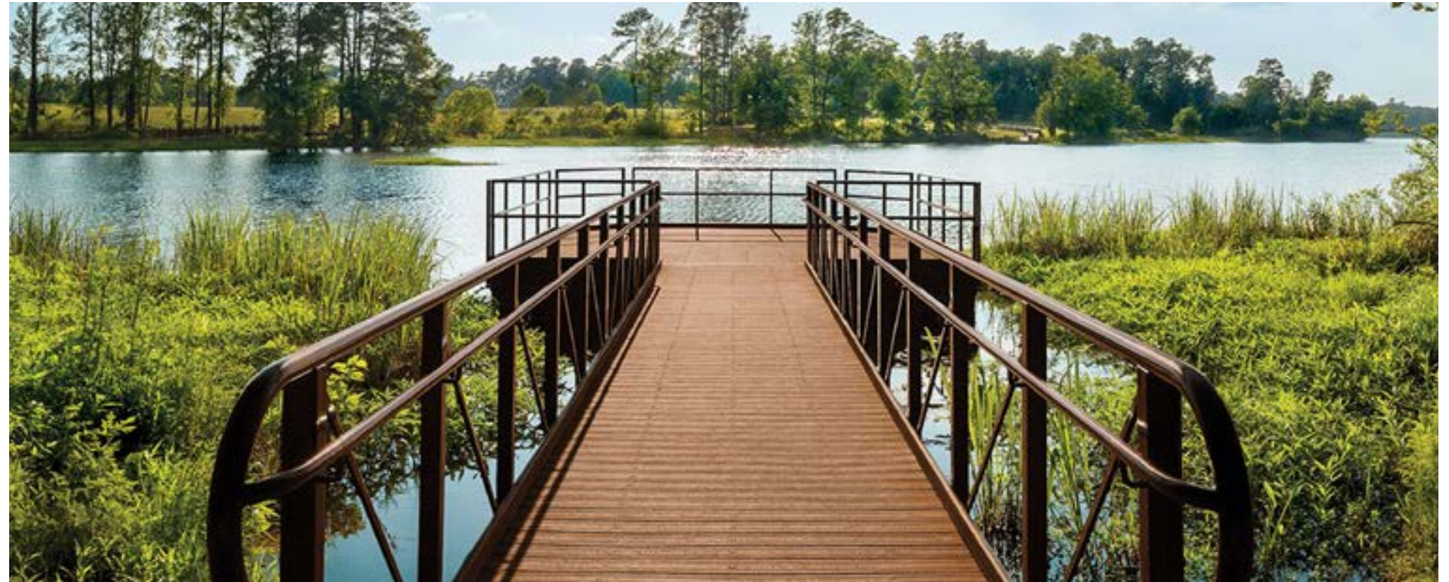
composite decking pier
