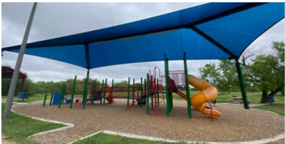
playground with fabric shade canopy
